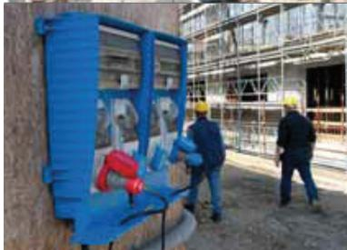
The cable clamp groove avoids the possibility that the plug can be torn from the board when it is wall mounted.
